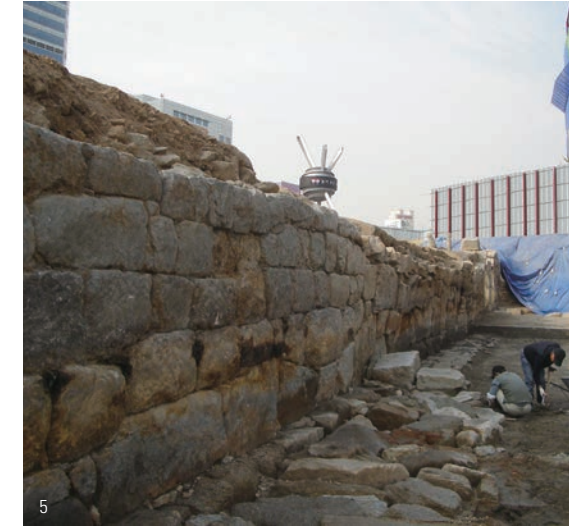
5. Excavation for the construction of Dongdaemun Design Plaza, where relics such as a twin-arched water gate and a projecting outwork were found.
